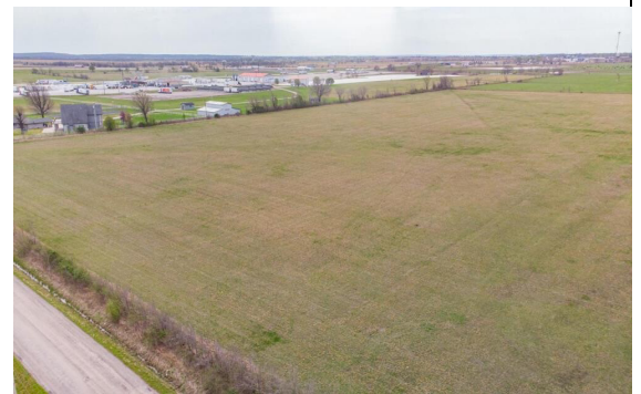
E. 310 Road — ODOT Major Collector, paved
