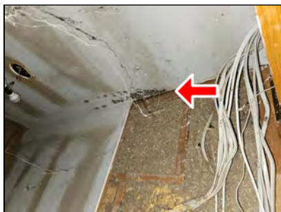
Stairway to basement.
