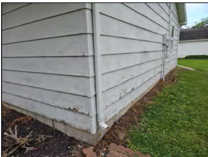
West side of the garage
