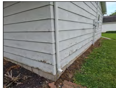
West side of the garage
