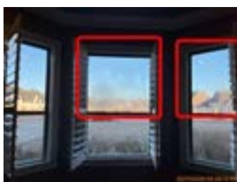
Downstairs front right bedroom
