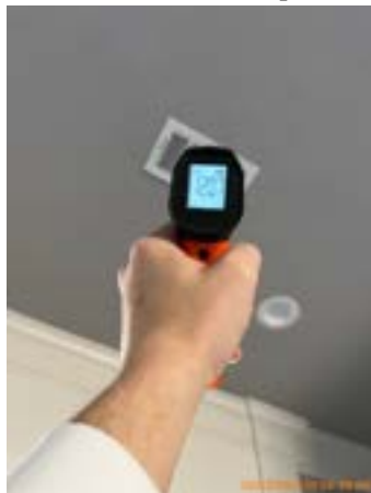
Downstairs main supply
