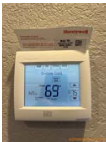
Downstairs front right Bedroom
