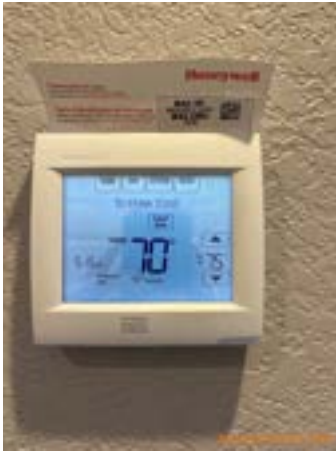
Downstairs front right Bedroom
