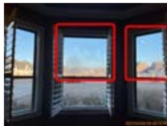
Downstairs front right bedroom
