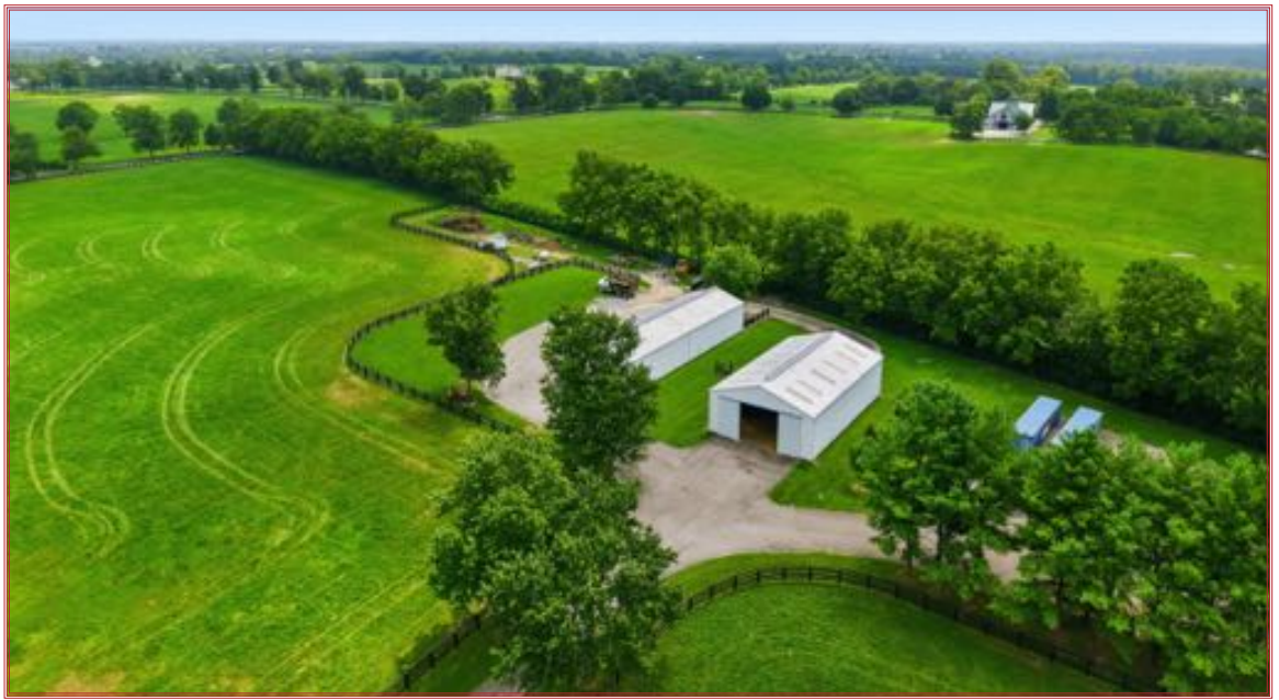
Storage and equipment buildings
